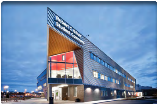
The new Student Commons - built to LEED® Gold standards - is one of the college's flagship buildings.
