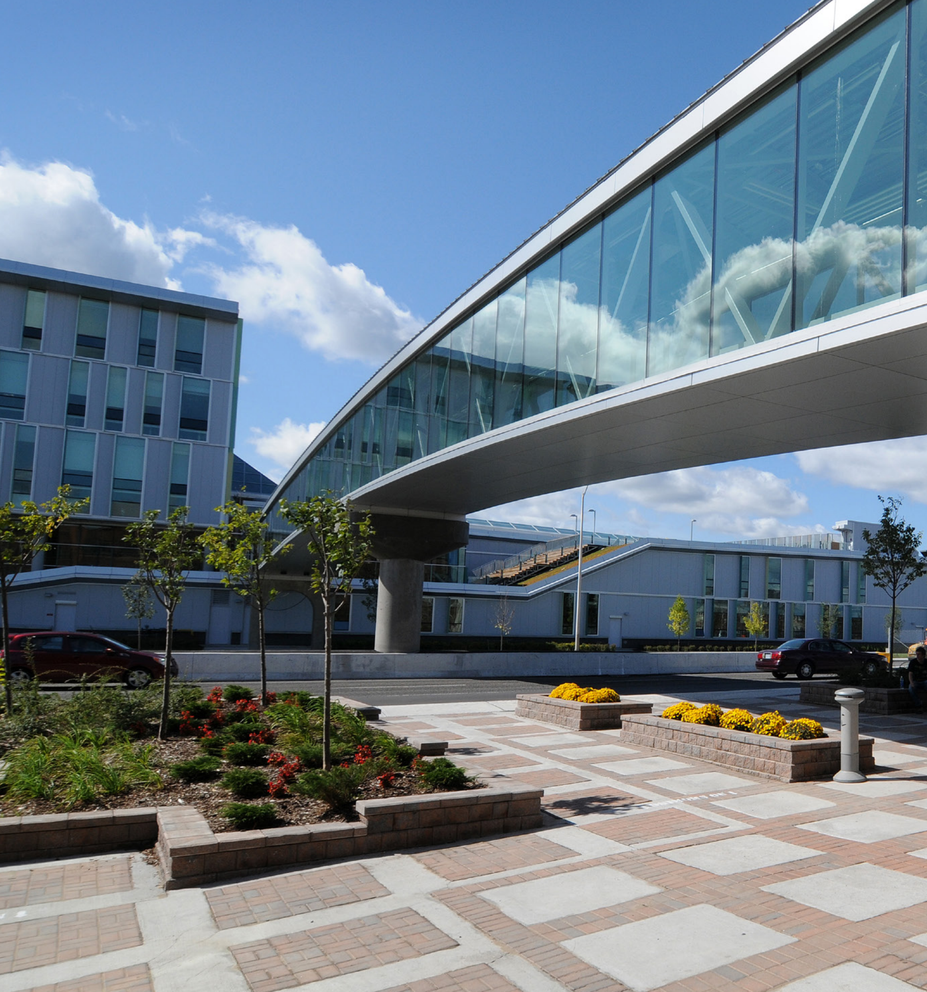
Bridge to the Algonquin Centre for Construction Excellence on the Ottawa Campus.
