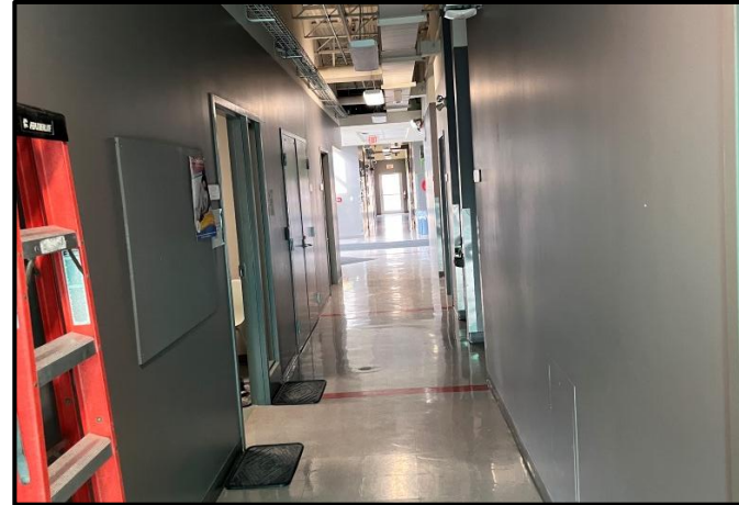
Photograph 2: Typical view of main corridor in Building Z.
