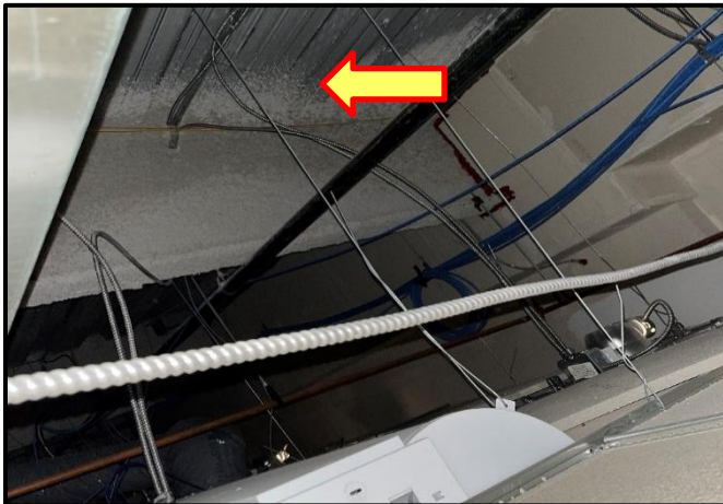
Photograph 3: View of non-asbestos containing sprayed fireproofing observed in ceiling spaces throughout.
