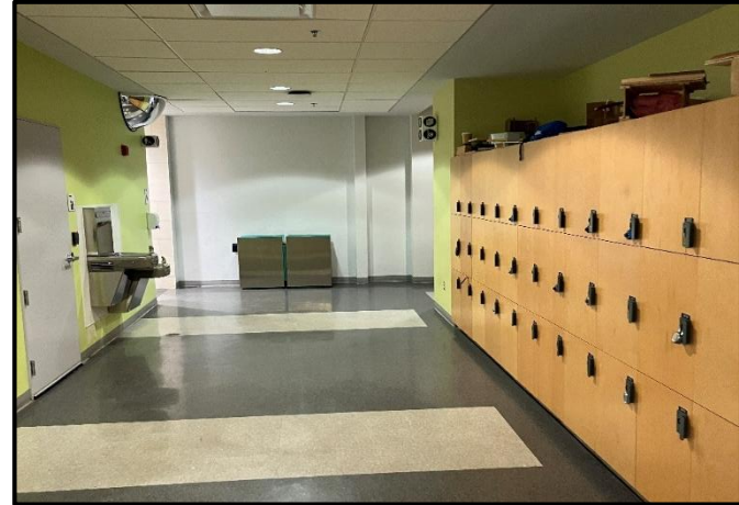
Photograph 2: Typical view of corridors within the building.
