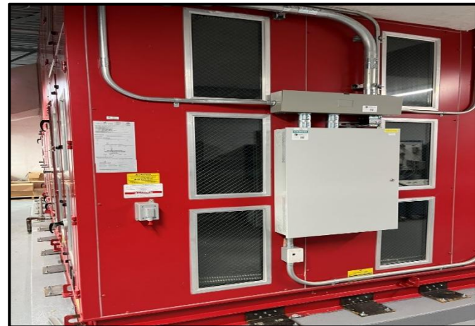
Photograph 8: View of air handling unit observed in the sixth-floor mechanical penthouse.
