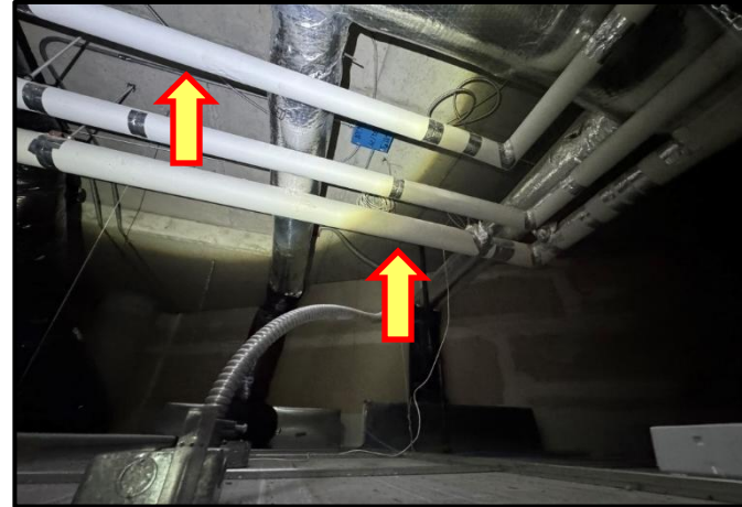
Photograph 2: View of non-asbestos fiberglass insulation observed in ceiling spaces throughout the building.
