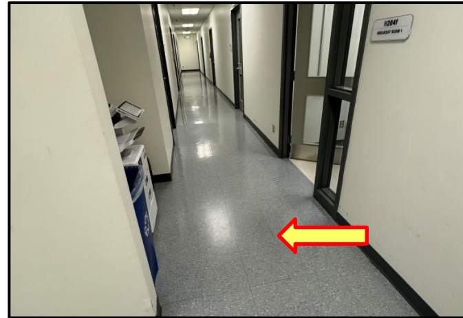
Photograph 10: View of non-asbestos containing 12"x12" Grey vinyl floor tiles.
