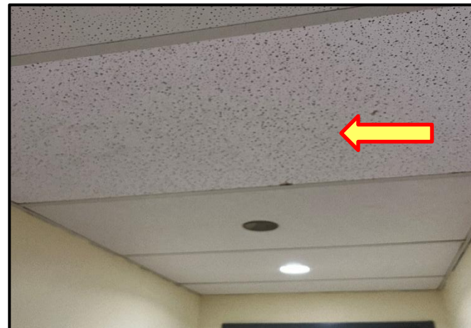
Photograph 2: View of non-asbestos containing acoustic ceiling tiles observed throughout the building.
