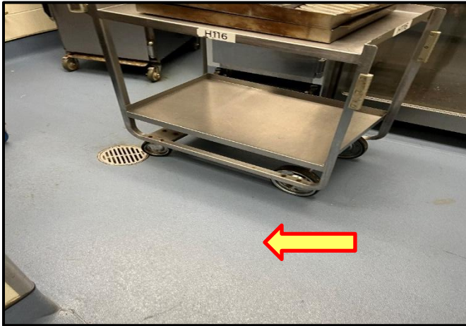
Photograph 5: View of non-asbestos containing sheet vinyl flooring observed throughout the building.
