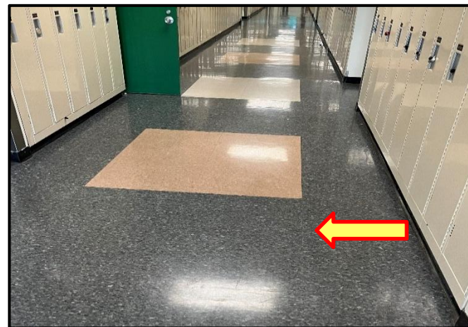
Photograph 4: View of non-asbestos containing 12"x12" vinyl floor tiles.
