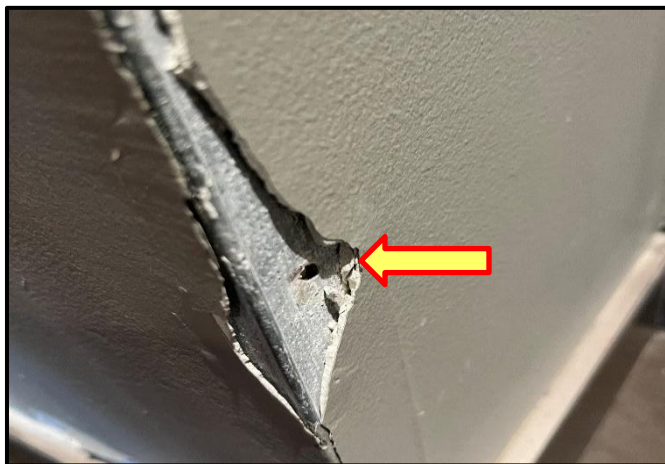
Photograph 3: View of non-asbestos containing drywall joint compound observed throughout the building.
