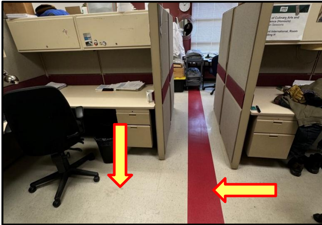
Photograph 9: View of non-asbestos containing 12"x12" vinyl floor tiles.
