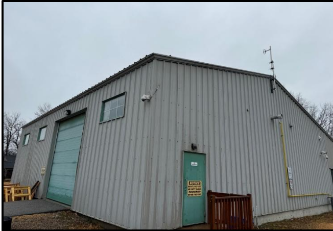
Photograph 9: Typical view of the exterior of Building B (Carpentry Workshop).
