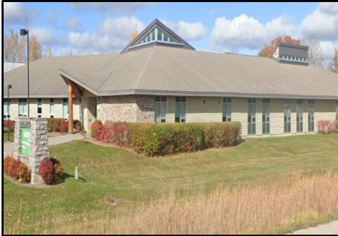
Photograph 1: Typical view of the exterior of Building A.
