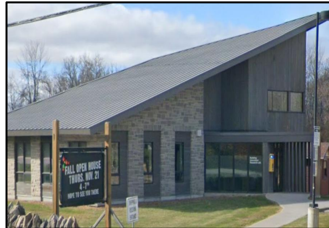
Photograph 12: Typical view of the exterior of the Residential Living Lab building.
