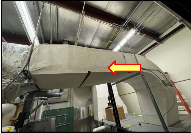
Photograph 5: View of non-asbestos fiberglass insulation observed on ductwork.
