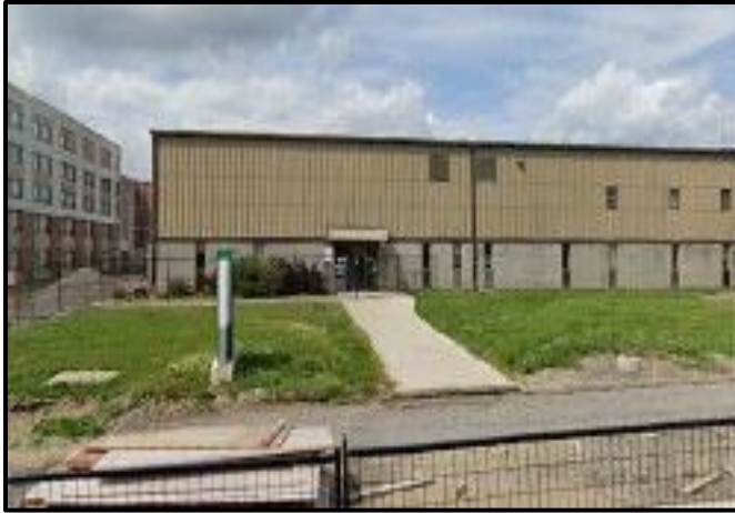
Photograph 1:View of the exterior of the building.
