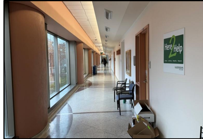
Photograph 2: Typical view of corridors on the first-floor of the building.
