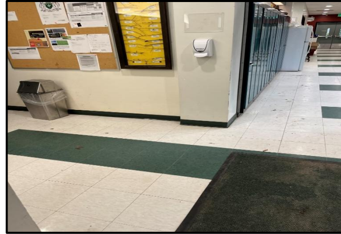
Photograph 2: Typical view of the corridors observed throughout the building.
