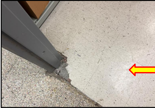
Photograph 13:View of asbestos-containing 12"x12" white vinyl floor tiles with black and grey streaks observed in Room A2114.
