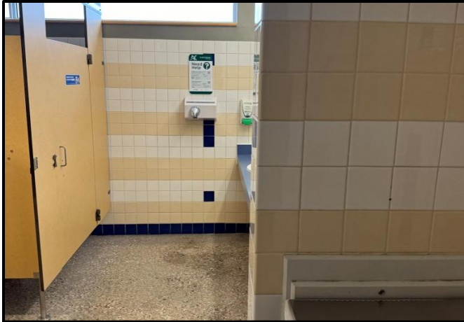
Photograph 5: Typical view of the washrooms observed throughout the building.
