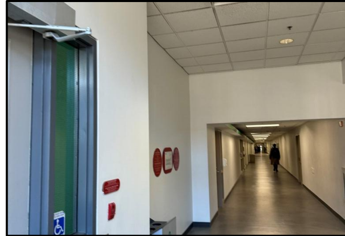
Photograph 2: Typical view of the first-floor corridor.
