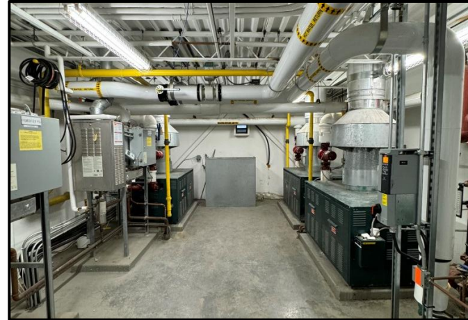
Photograph 6: View of mechanical penthouse B.
