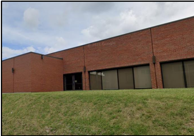
Photograph 1: Typical view of the exterior of the building.
