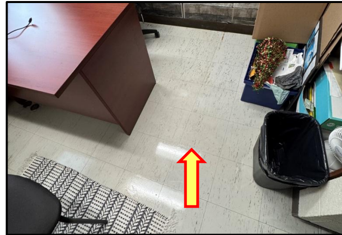
Photograph 2: View of asbestos-containing 12"x12" grey vinyl floor tiles.
