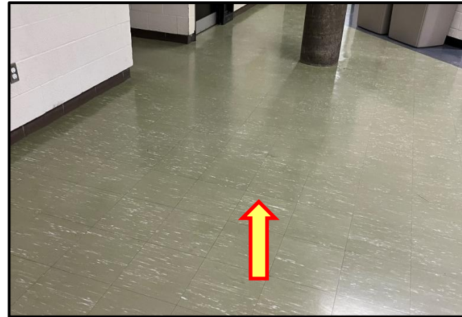
Photograph 10: View of asbestos-containing 12"x12" green vinyl floor tiles.
