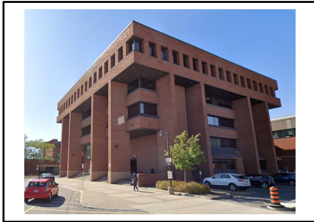
Photograph 1: View of the exterior of the building.
