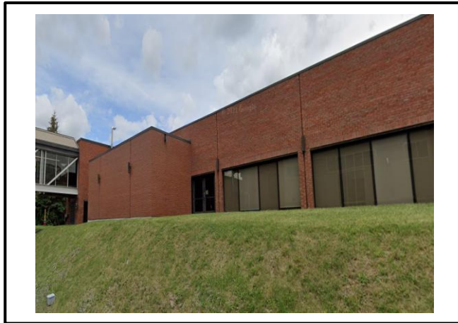
Photograph 1: View of the exterior of the building.
