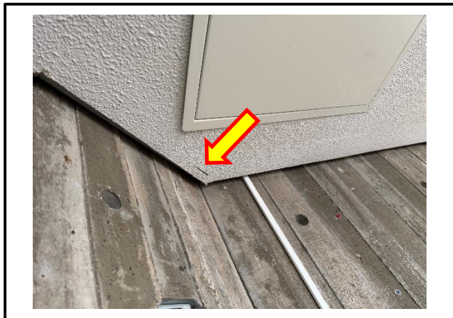
Photograph 13: View of the damaged asbestos-containing ceiling stipple observed in Room B414.
