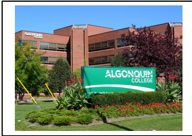
Photograph 1: View of the exterior of the building.
